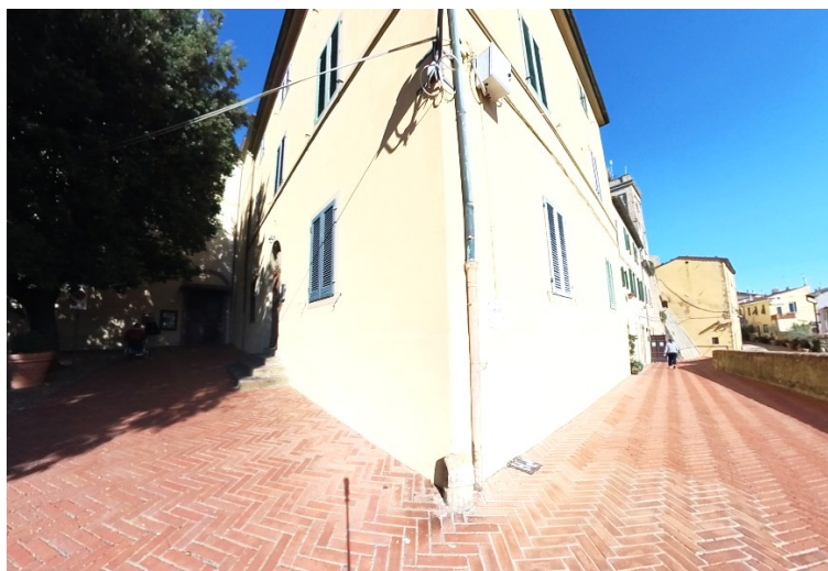
Figure 18 path on the left towards the side entrance Church of S. Maria Assunta
